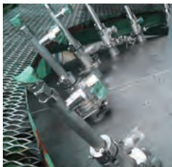
Nozzle installation in the cooling tower
