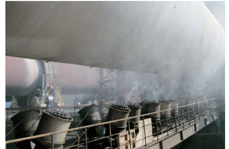
Industrial cooling system
