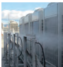
COOLSAVE-D fog cooling for air-conditioner outdoor units
