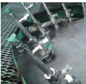
Nozzle installation locations in a cooling tower
