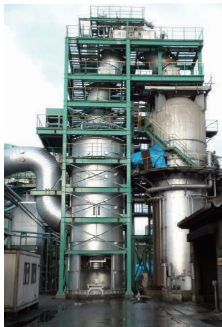
Gas cooling tower (Photo courtesy of JX NIPPON TOMAKOMAI CHEMICAL CO., LTD.)
