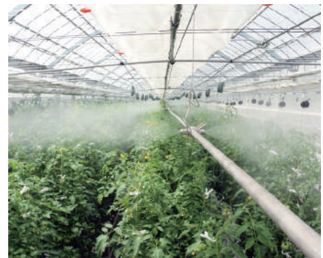
CoolPescon® CH greenhouse cooling and humidification system
