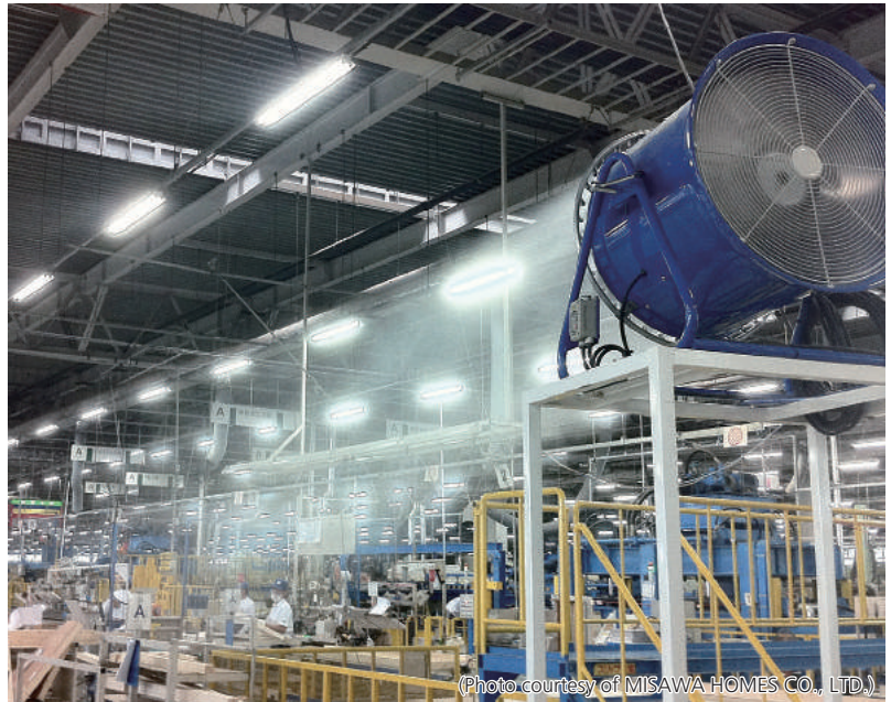
COOLJetter® Dome energy-efficient, large-space cooling system
