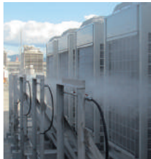
COOLSAVE-D fog cooling for air-conditioner outdoor units
